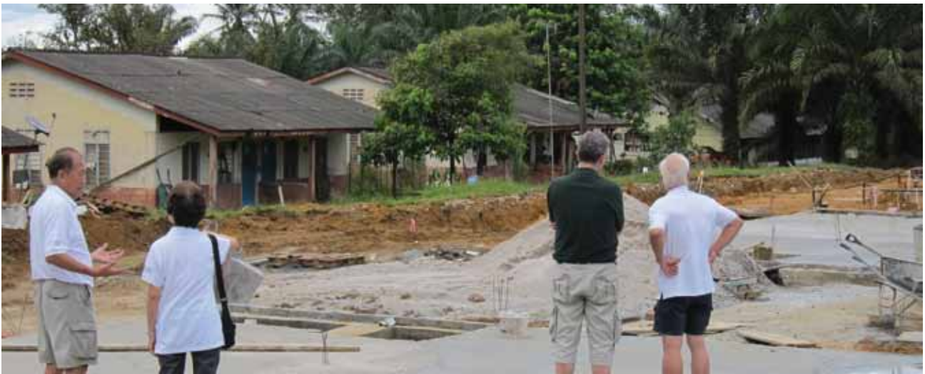
■ Labour Lines & Staff Quarters under construction – Narborough Estate
