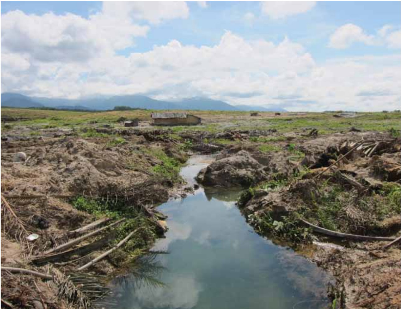
■ Preparation of drains during replanting – Hibernia Estate
